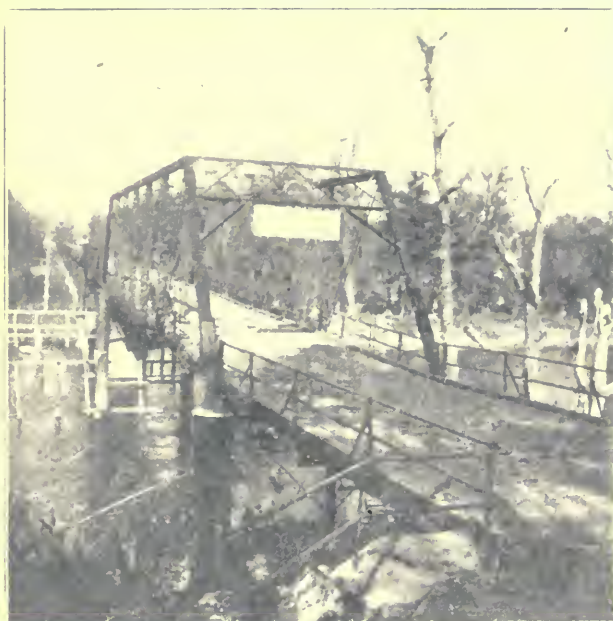
NEW STEEL BRIDGE ACROSS TAR RIVER AT GREENVILLE
